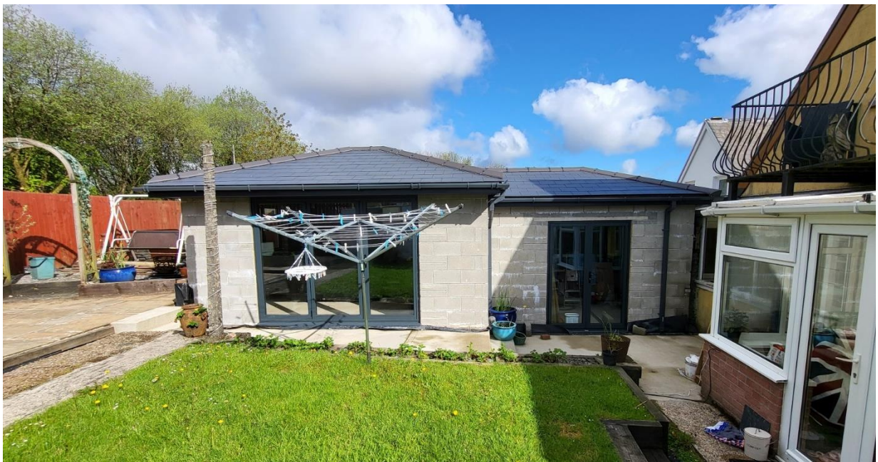
Figure 1.1 Photo of garden room
