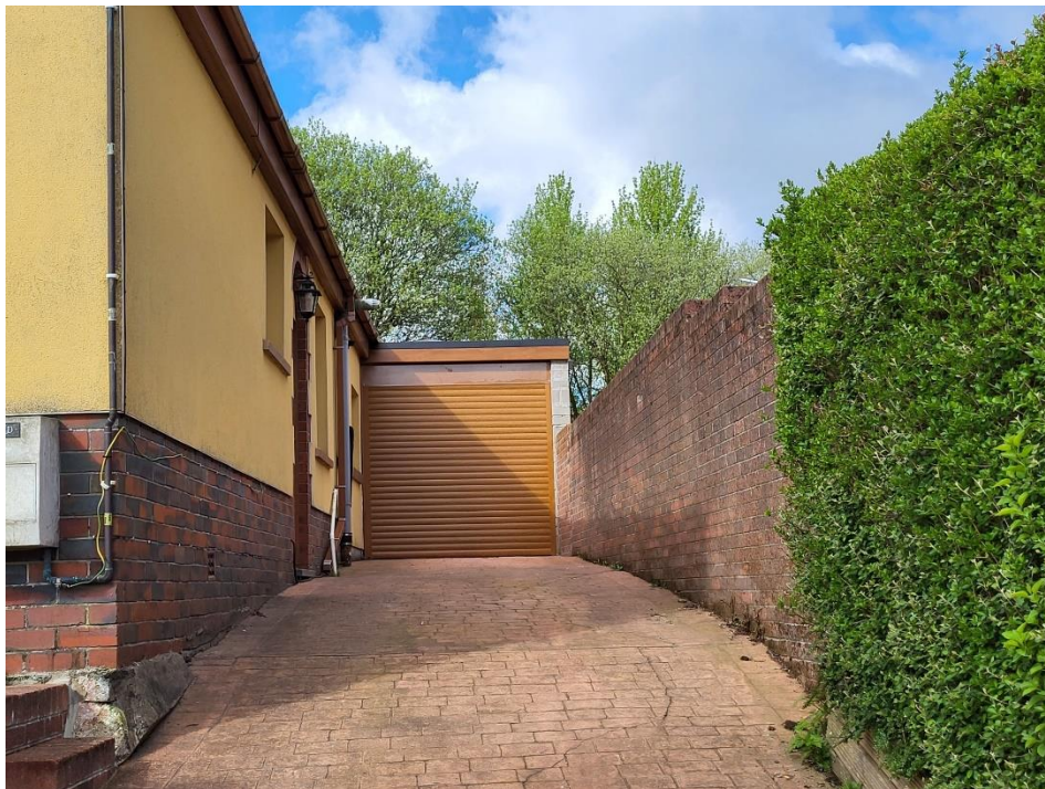
Figure 1.11 Photo of front elevation of garage from Badminton Grove
